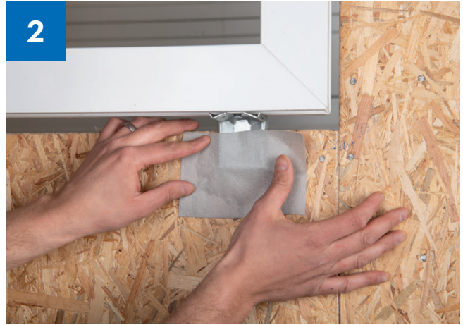
> If necessary, apply over the mounting bracket.
