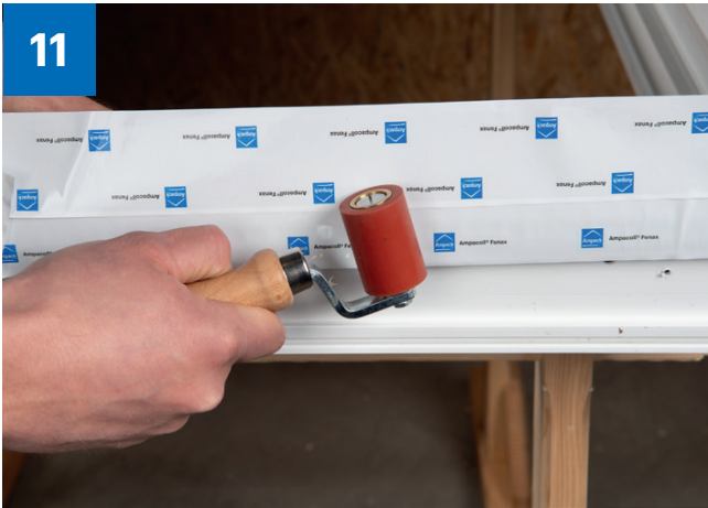
11 > Roll up the window skirt all around.
