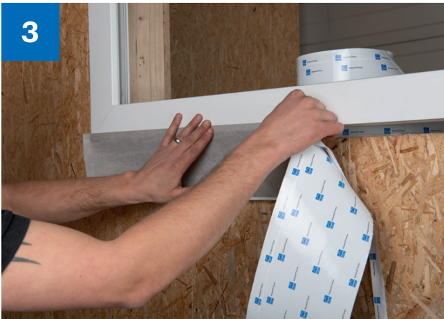
> Start application at the bottom.
