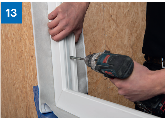
13 > Initial situation: Built-in window frame with prefabricated adhesive tape skirt. Decide whether to start the installation on the inside or outside depending on the local conditions or the specifications of the planner (consider weather conditions and construction progress).
