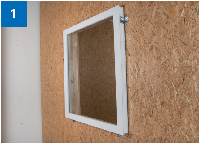
> Externally mounted frame.
