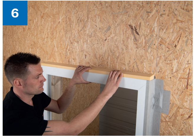
> Mount the insulating wedge on the upper side.
