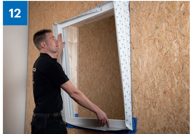
12 > Mount the window frame professionally in the wall opening.
